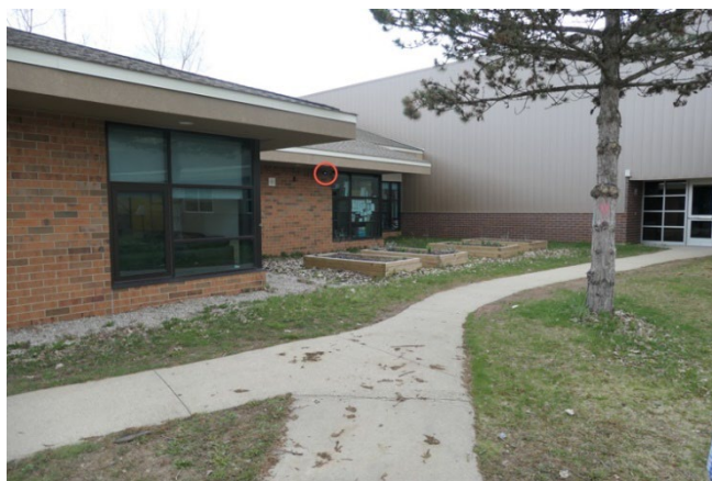
Figure 28: North Courtyard Horn
