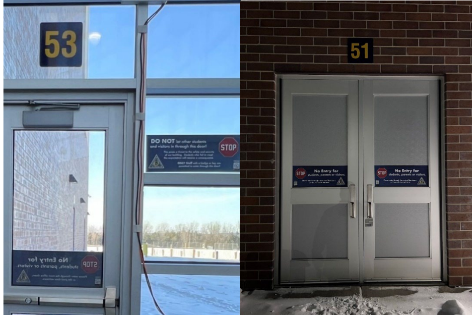
Figure 11: Doors Not to Be Used for Entry
