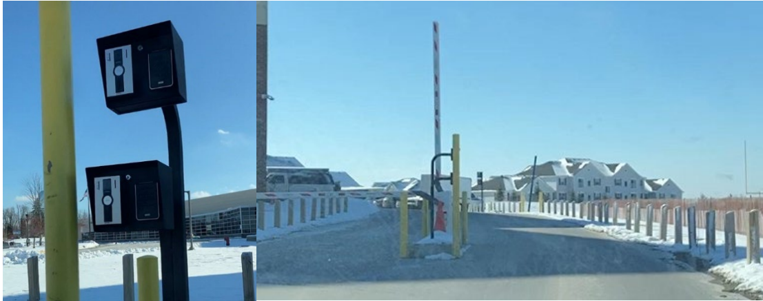
Figure 8: Perimeter Vehicle Barrier
