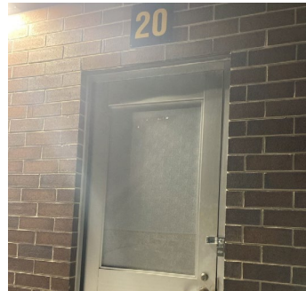
Figure 39: Door 20 with Padlock on Exterior
